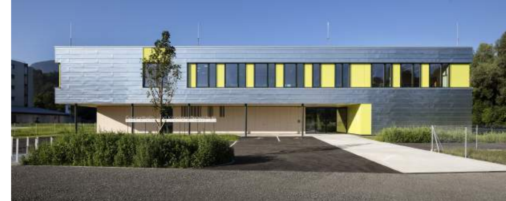
Schimmernde Alu-Blechfassade - fotocredit by Andrew Phelps
